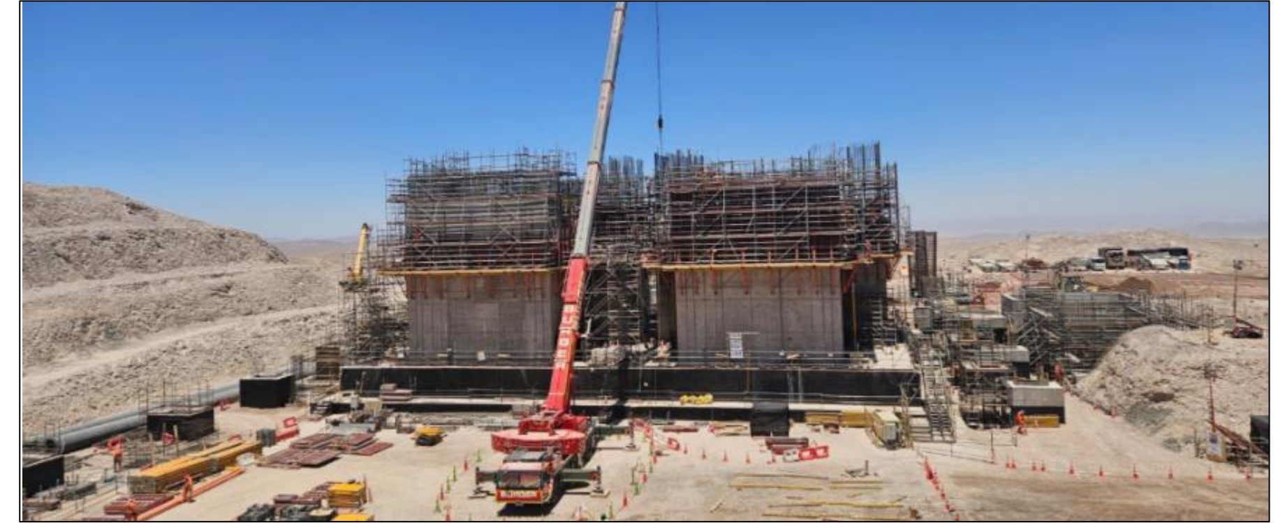
Image: Concrete pouring, main concentrator site
