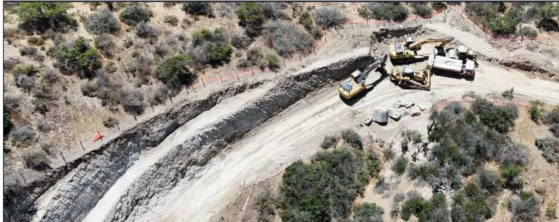
Image: Access road construction, ahead of installing pipeline (lower section)
