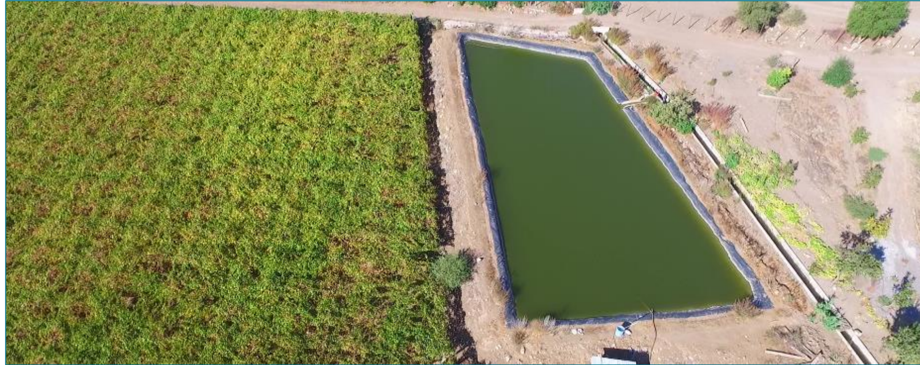
Image: Water storage ponds for local communities, built under Confluye Programme (part of Somos Choapa)
