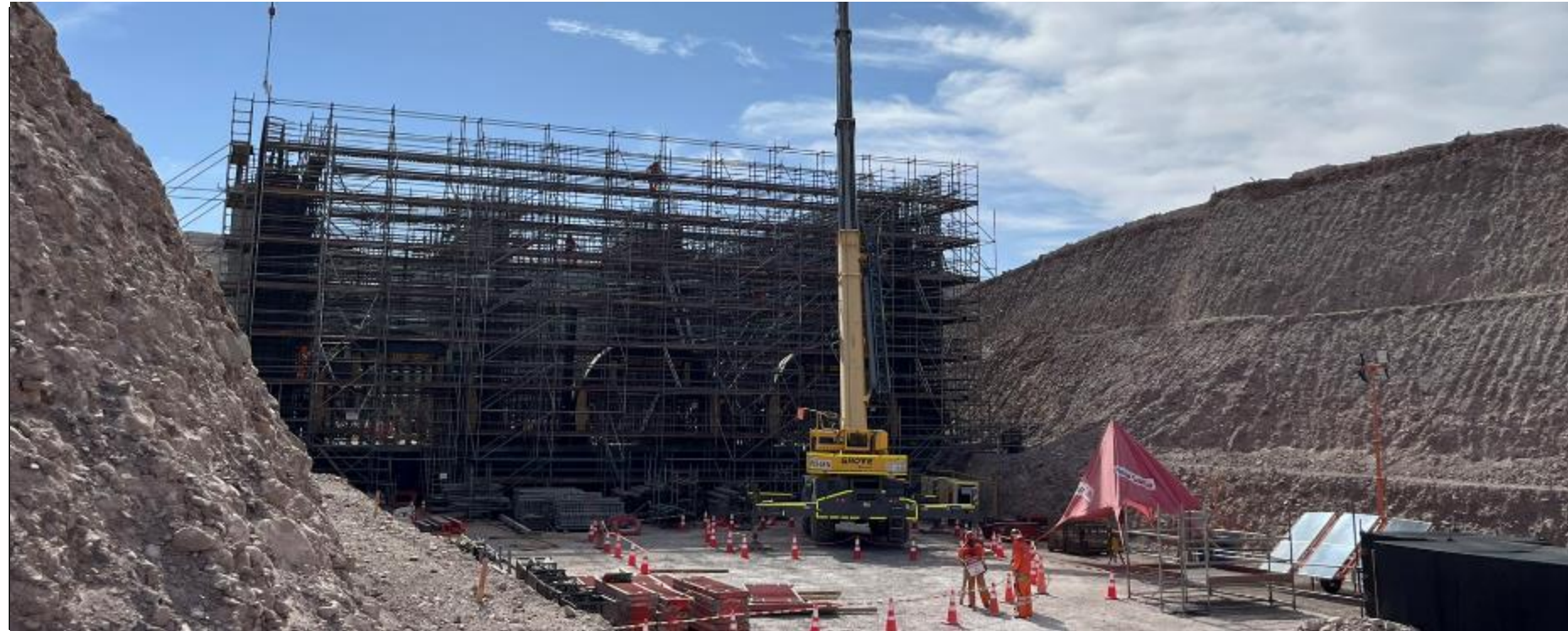
Image: Installation of ore rehandling tunnels, main concentrator site
