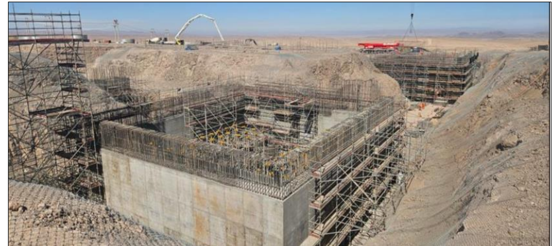
Image: Primary crusher foundations, adjacent to Esperanza Sur pit
